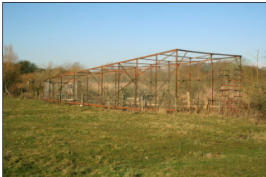
The newly constructed Heligoland trap in 2007
